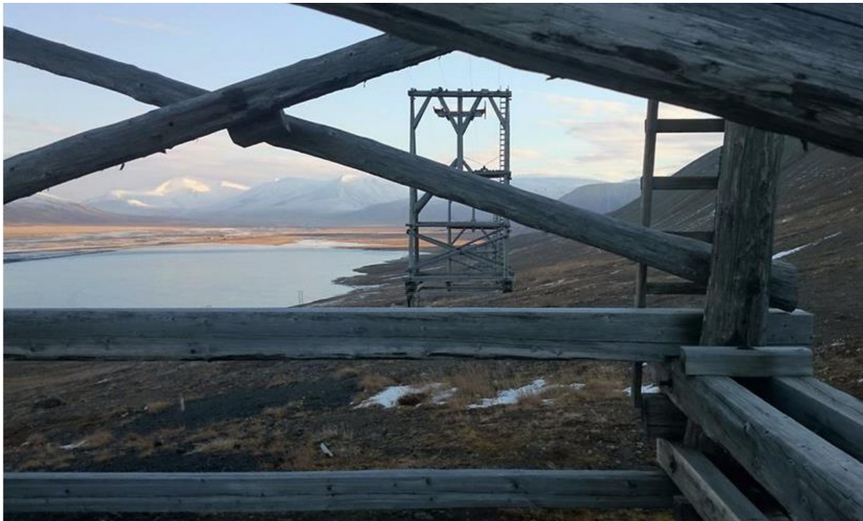
Figure 3. Cable way timber trestles in Longyearbyen. Photo: Anatoly Sinitsyn, NTNU
