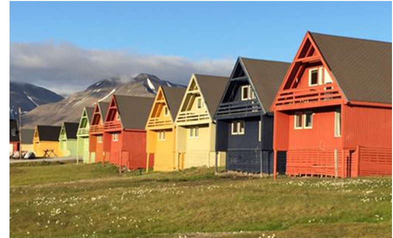
Buildings in Longyearbyen threatened by thawing permafrost. Photo: L. Iversen, NERSC
